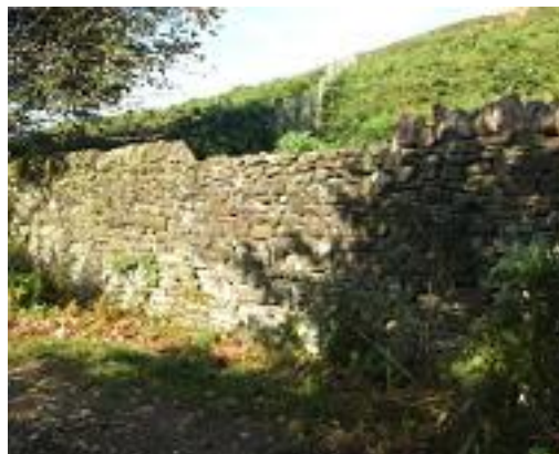
Photograph 2: Beeley Hilltop, a BOAT in Derbyshire where coping stones were removed from the wall by green laners to fill ruts in the route. September 2013
