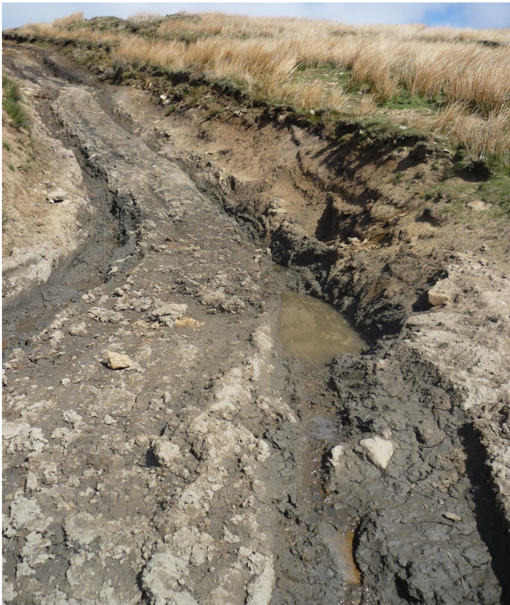
Deadman's Hill after repair
